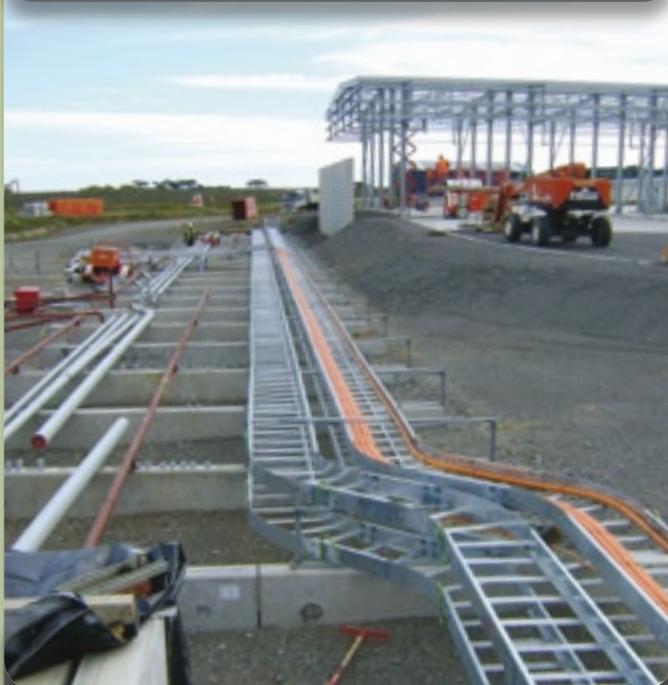
Pipe trays will carry 300km of cable around the Kupe Production Station
