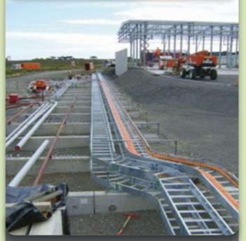
Pipe trays will carry 300km of cable around the Kupe Production Station
