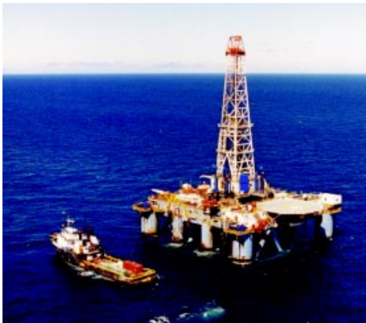
Offshore semi-submersible drilling unit.
