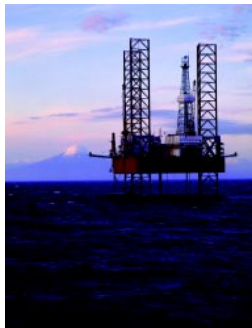
JFP-11 jack-up drilling unit.
