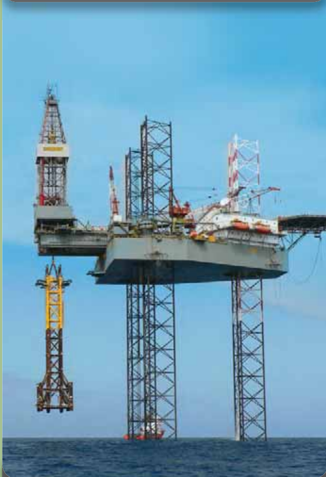
Ensco-107 drilling rig installing the Kupe production platform
