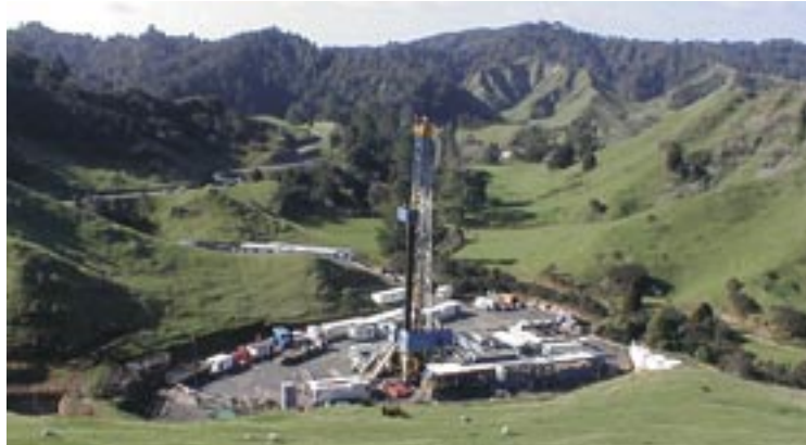
Tuihu-1A drilling in progress
