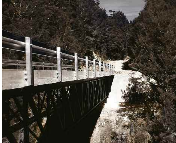
First major bridge at Pike
