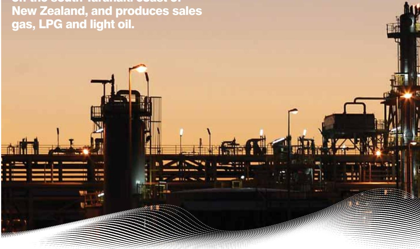
**The development of the Kupe Central Field Area comprises three production wells, a normally unmanned offshore platform, a 30km pipeline and associated umbilical to shore, an onshore production facility near Hawera, and oil storage facilities at New Plymouth.**
